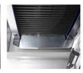
**Collecting the condensation**The large tray allows the correct flow of condensate in order to keep the floor of the blast chiller dry.
